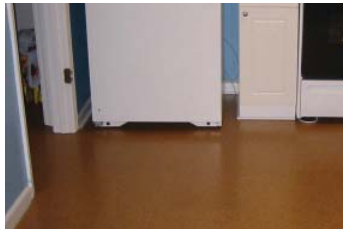
Sustainable materials were used throughout the home. Including: cork, bamboo, wheat board flooring instead of particle board and corrugated metal ceiling.
